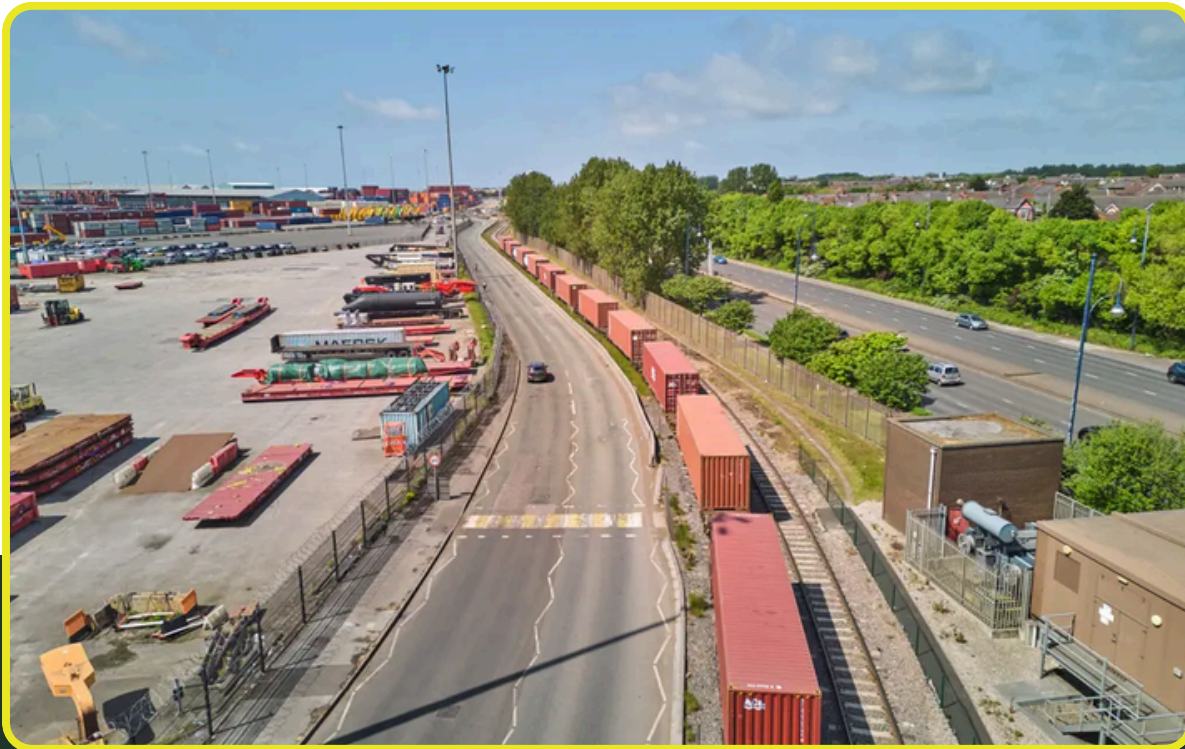
Port of Liverpool Rail Terminal, credit: Peel Ports
