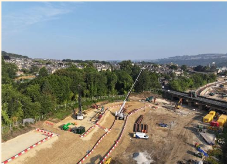
Shipley Depot underway
