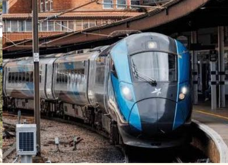
25% of TRU route electrified
