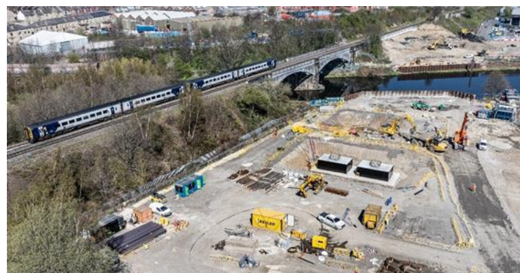
Aerial View of Baker Viaduct Piers 5 to 8
